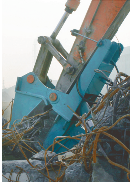
安装完毕 Finished installation
