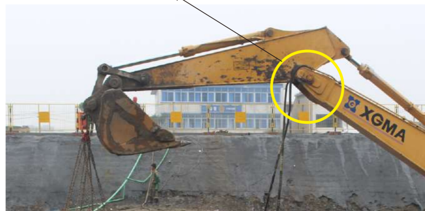
液压油管分离和安装部分 Hydraulic pipe separation and installation part
